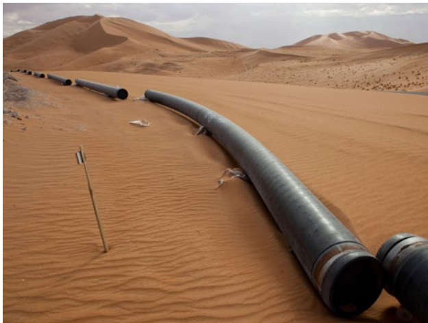
Pipeline construction in the Sahara desert. © Richard J Greenman / Alamy Stock Photo
